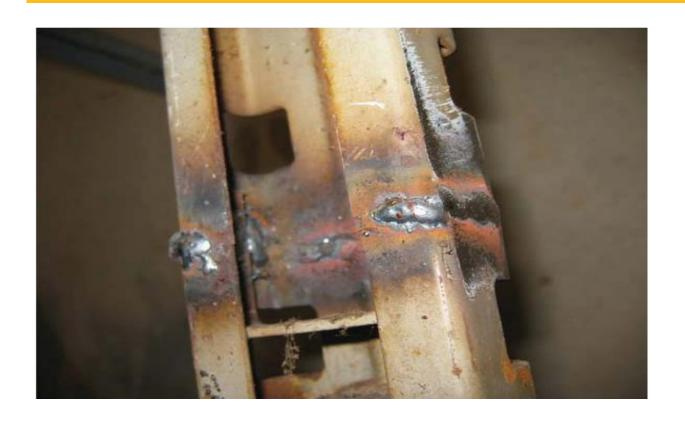
The capacity and/or safety of frames, and beams can be adversely affected if they are structurally modified e.g. cut down, spliced or welded
